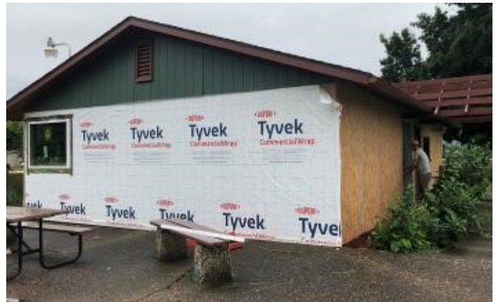
Exterior work was completed in the Fall of 2022 through the State's major maintenance fund, by the State Historical Society of Iowa. The Museum building received new windows, doors, and siding. Though the color remained the same, the structure has been much improved.
